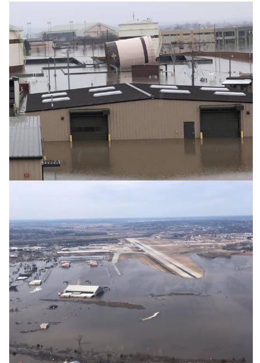
Flooding at Offutt AFB, NE (2019)
