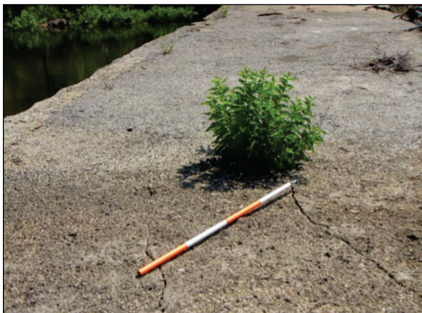
Figure H-4. Concrete cracking on crest (Ellithy, Rivera-Hernandez, and Abraham 2015).
