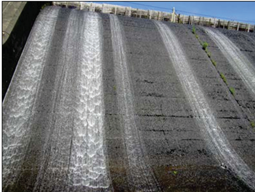
Figure H-7. Eroded concrete floor on spillway outlet (Landers et al. 2015).
