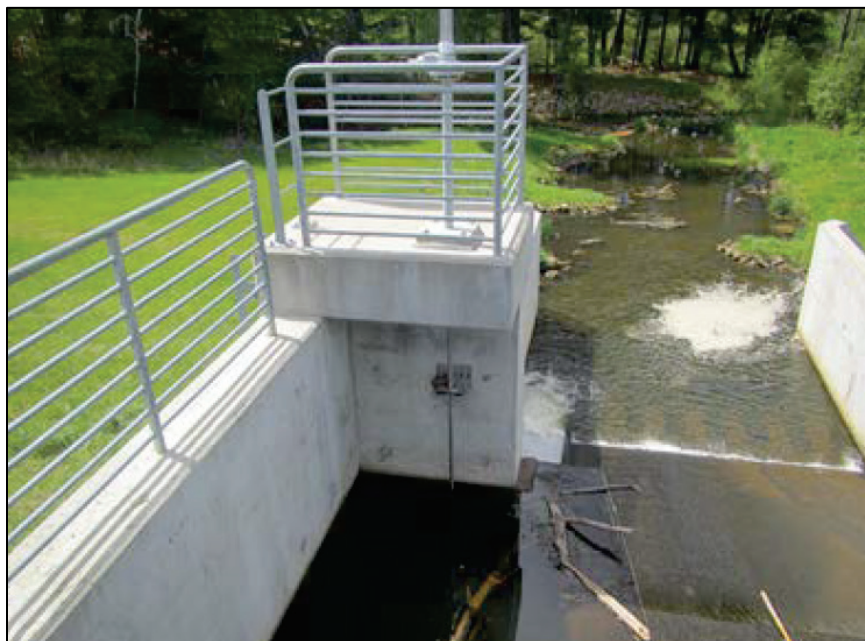
Figure H-2. Debris in inlet structure (Quinn et al. 2016).
