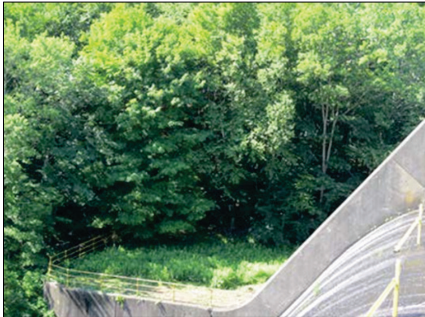
Figure H-5. Heavy vegetation on the downstream slope (Landers et al. 2015).
