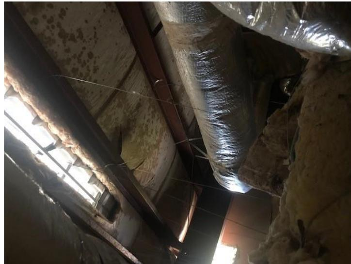
**Attic-** Roof leaks are causing moisture to collect in the insulation and damage ceilings.
