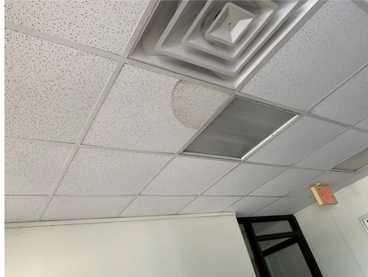
**Ceiling-** Acoustical Tiles show water damage.
